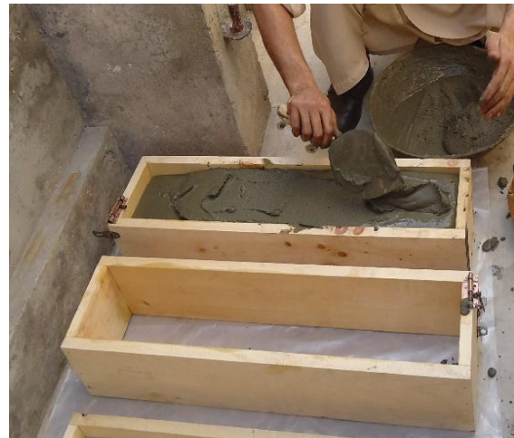
Figure 2: Pouring of ECC into the molds
